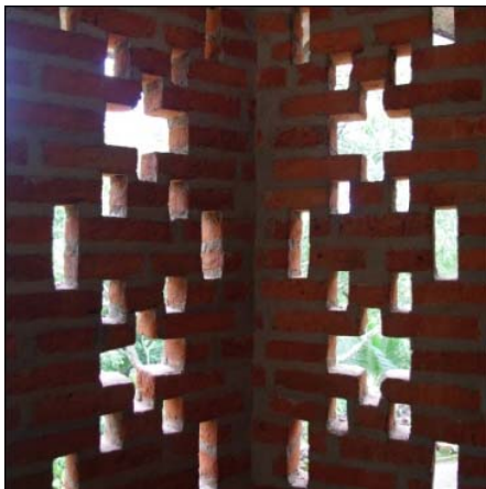
Brick Jaali for light and ventilation
